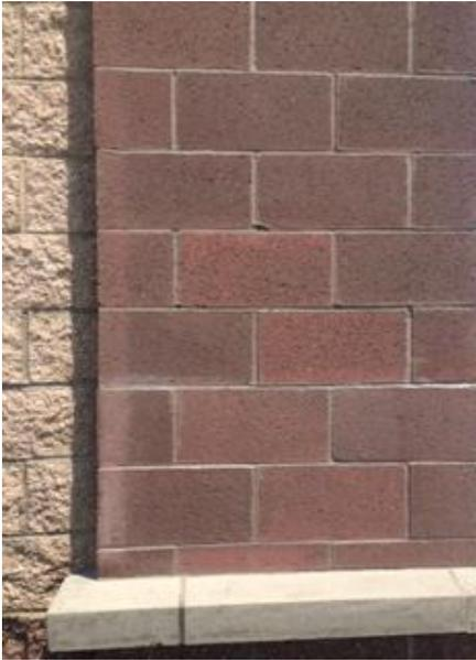
*Designers should understand the appearance issues with smooth-face concrete masonry walls.*
